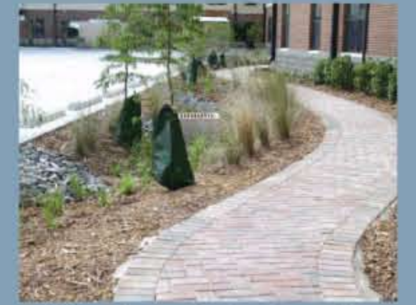
Bioswale near pedestrian walkway
