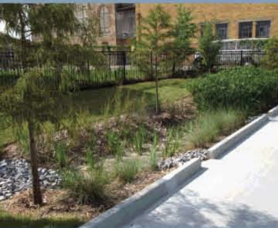
Site completion of the bio-swale.
