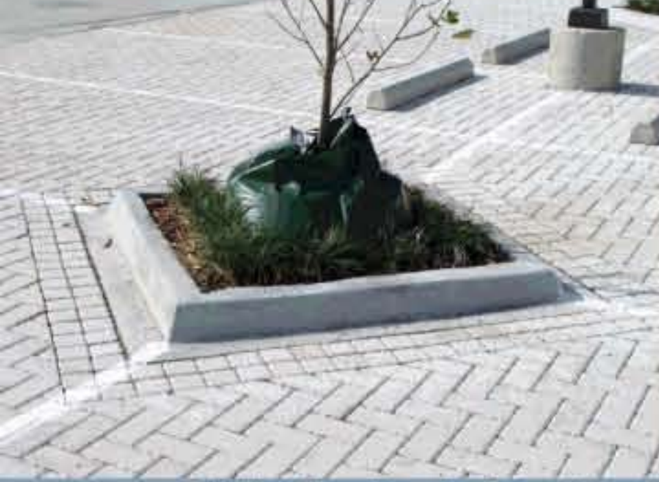
CMU soil parking lot for residents.
