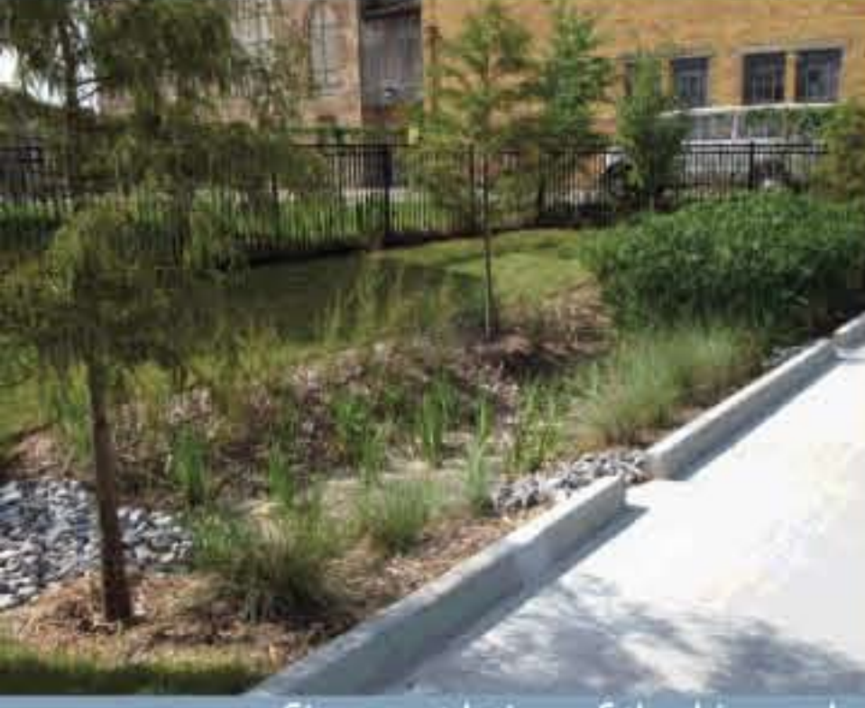
Site completion of the bio-swale.
