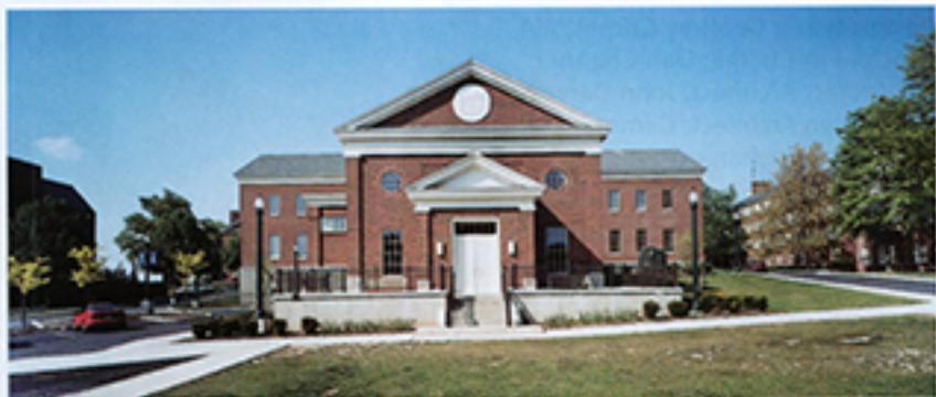
Entrance to recital hall lobby
